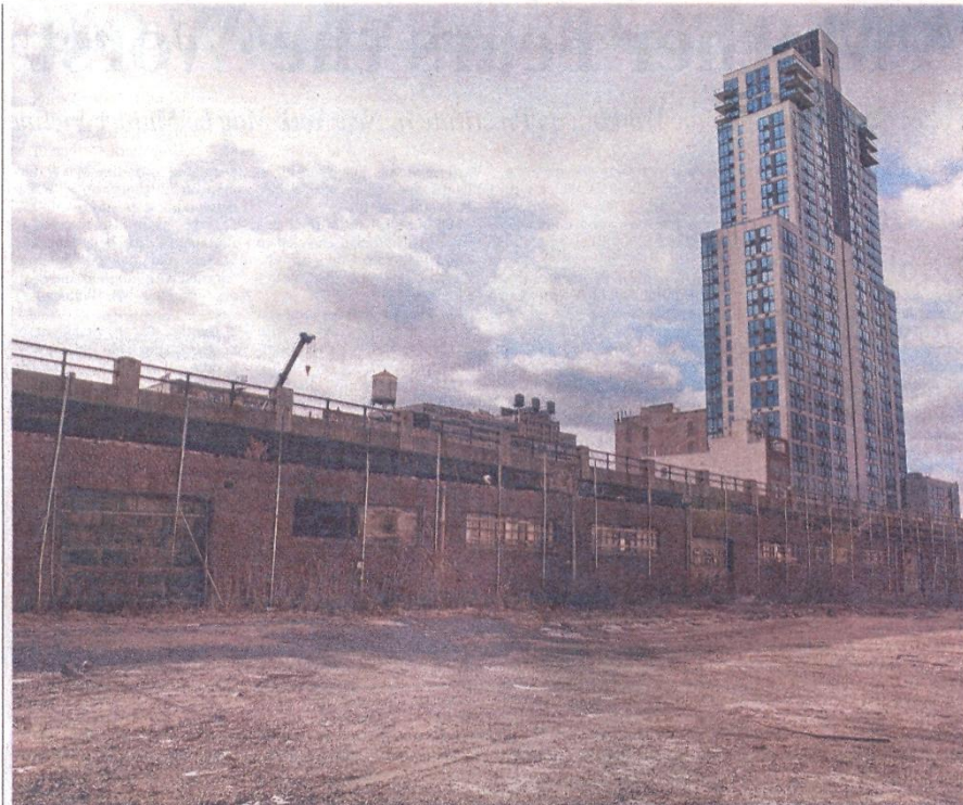
Development firm Related Cos. is awarding a contract to demolish a 60,000-square-foot building as part of work on the West Side rail yards, above.
